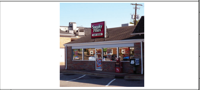
PREVIOUS SNEAKY PETE'S FRONT FACADE & SIGN
