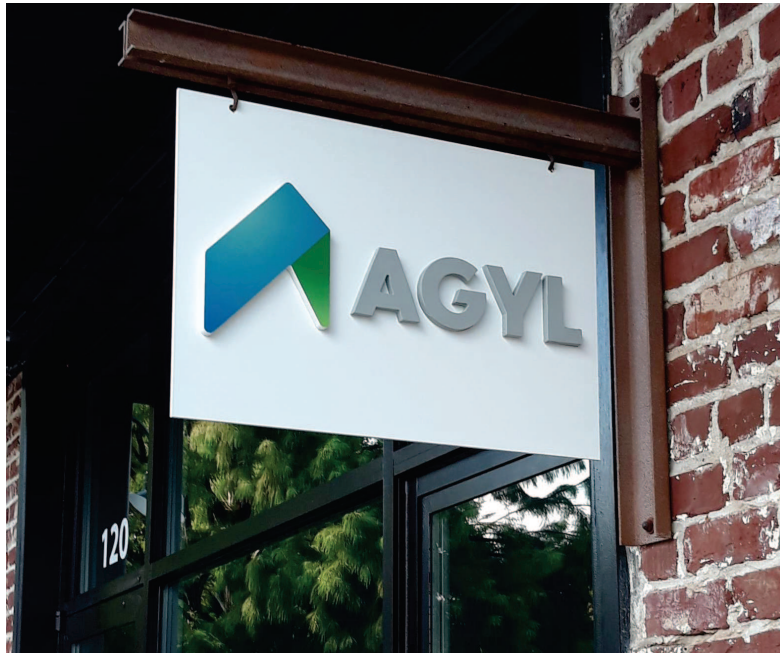
Sign showing similar construction to proposed sign with Aluminum Backer and PVC Copy
