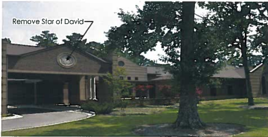
Existing Building – 3100 Overton Road
