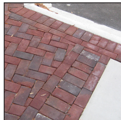
Brick at Sidewalk Corners
