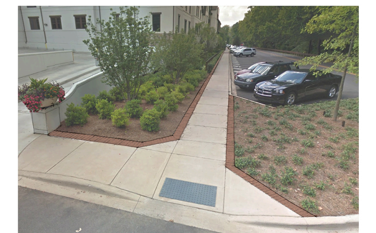
ADDED BRICK BORDER AT SIDEWALK
