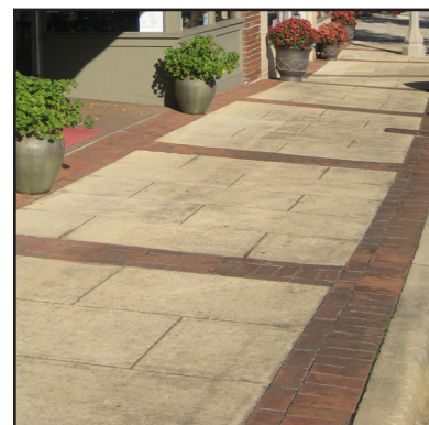
Scored Buff Concrete with Brick Bands
