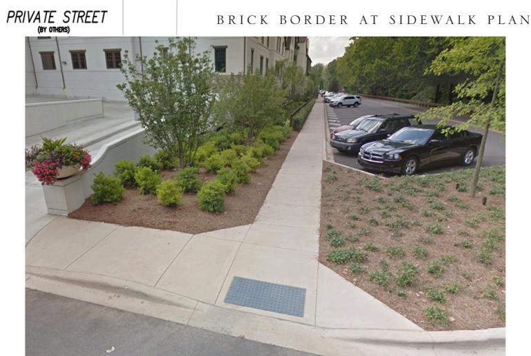
EXISTING CONDITIONS AT SIDEWALK
