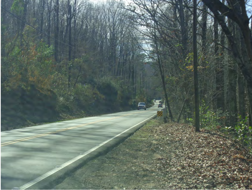
Figure 4: Difficult Sidewalk Installation – Old Leeds Road from Crosshill Road to Cherokee Road
