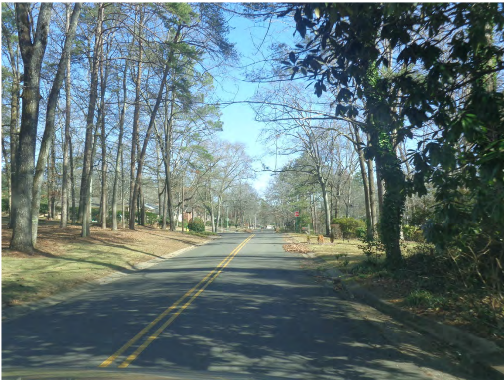
Figure 2: Easy Sidewalk Installation – Locksley Drive from Wheatherton Drive to Dunbarton Drive
