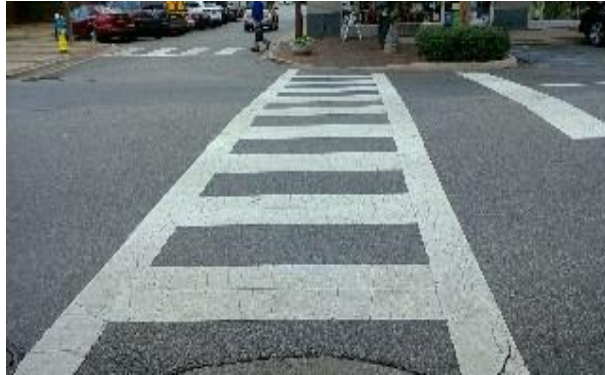
FIGURE 5: COMPLIANT CROSS WALK
