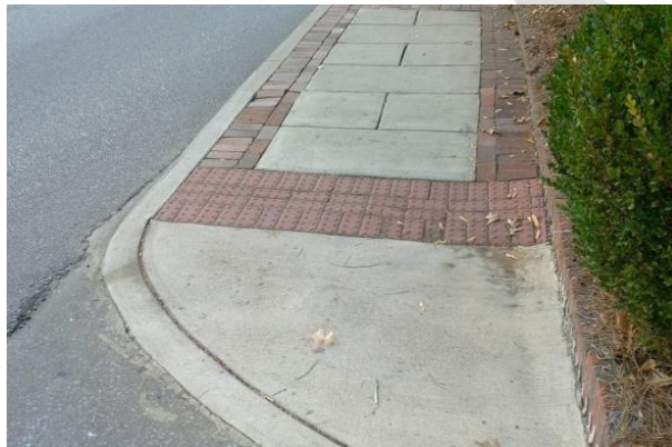
FIGURE 3: COMPLIANT CURB RAMP
