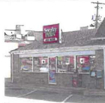
PREVIOUS SNEAKY PETE'S FRONT FACADE & SIGN
