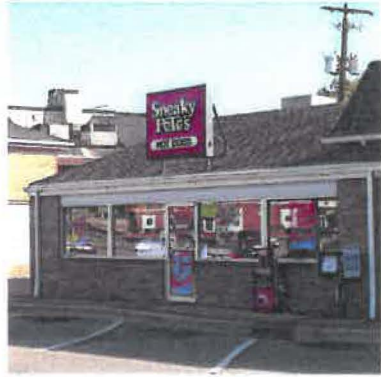
PREVIOUS SNEAKY PETE'S FRONT FACADE & SIGN
