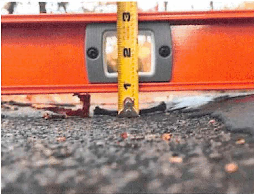
Photograph 10, Area 5: Rutting Depth of 0.75" (Surface Road Condition same as Area 1)
