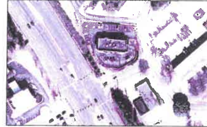
Aerial - 7 Office Park Circle
