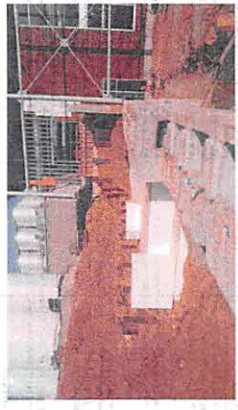
Figure 5.1.1 – Example View of EPS Backfill Behind Gravity Retaining Wall (From Author's Personal Photos)
