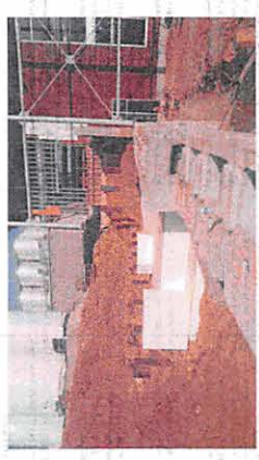
Figure 5.1.1 – Example View of EPS Backfill Behind Gravity Retaining Wall (From Author's Personal Photos)
