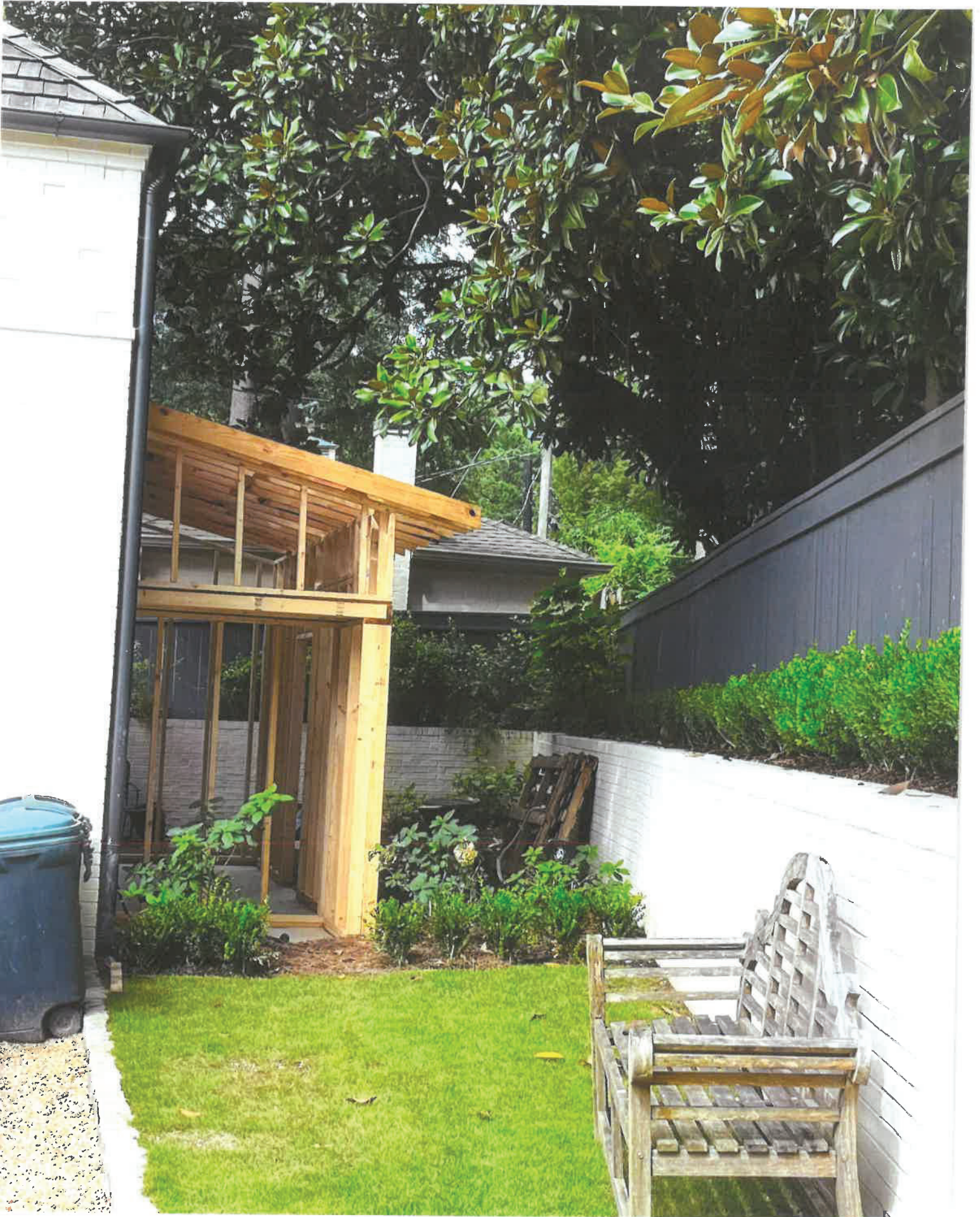
SIDE VIEW OF CLOSET ALREADY BEGUN
