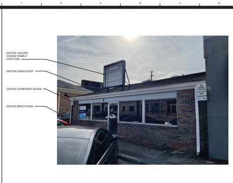
K7 EXISTING BUILDING STREET FACADE SCALE: 1/16" = 1'-0"
