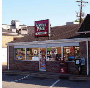
PREVIOUS SNEAKY PETE'S FRONT FACADE & SIGN
