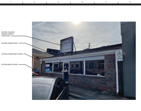
K7 EXISTING BUILDING STREET FACADE SCALE: 1/16" = 1'-0"
